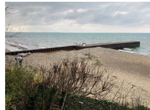
Whitewood Beach Pier (2023)
