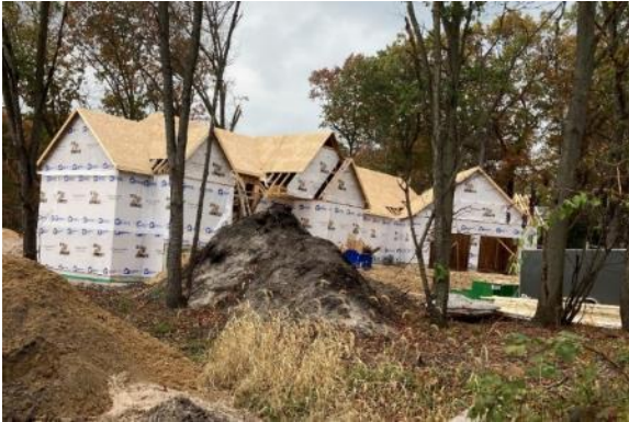
Golfmore Estates Construction Boom (2023)
