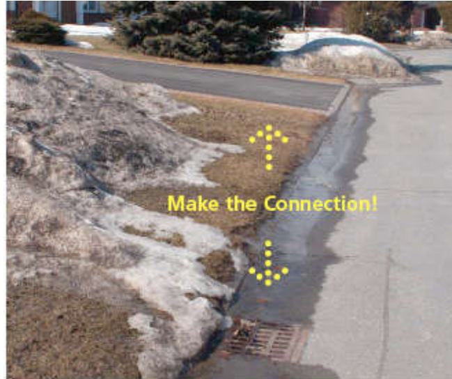
Storm drains carry road runoff directly to our rivers.
